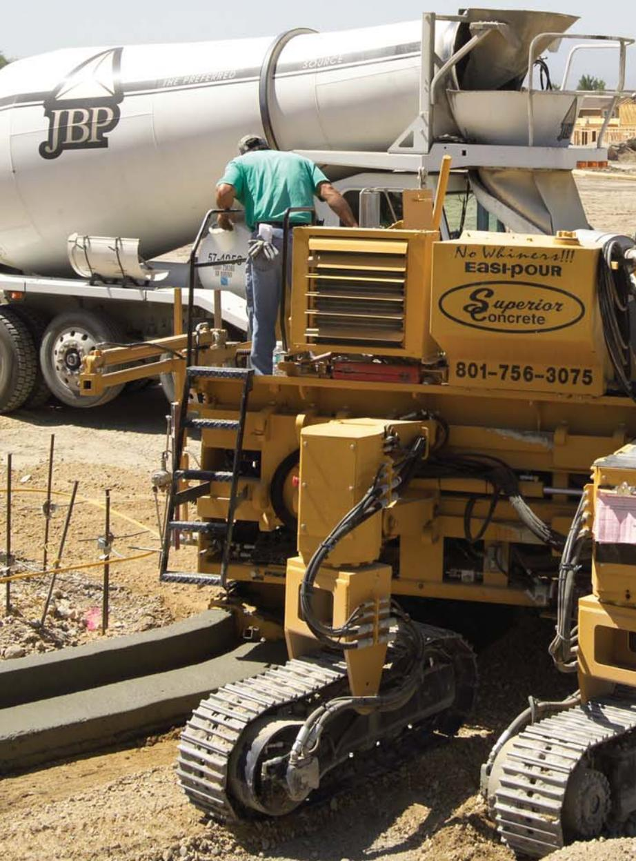
concrete in a mold, guided by a string-line sensing system also manufactured by Huron. The stringline system automatically ensures perfect steering and grade by incorporating five sensors — two steering, two grade, and one cross-level control. The 880 machine also comes with a grade trimmer with a standard width of 51 in. to trim high spots from the road surface.
