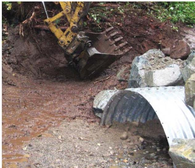
machine, building benches, doing nearly everything imaginable to get at the right angle for the job prior to using a tilting attachment. Now our equipment operators can just work from the road surface and use the PowerTilt to adjust the angle of the attachment instead of moving the entire excavator around.” Tony Holt, Equipment Operator agrees, “We had previously used a conventional bucket and thumb combination to complete our projects around the job site —
